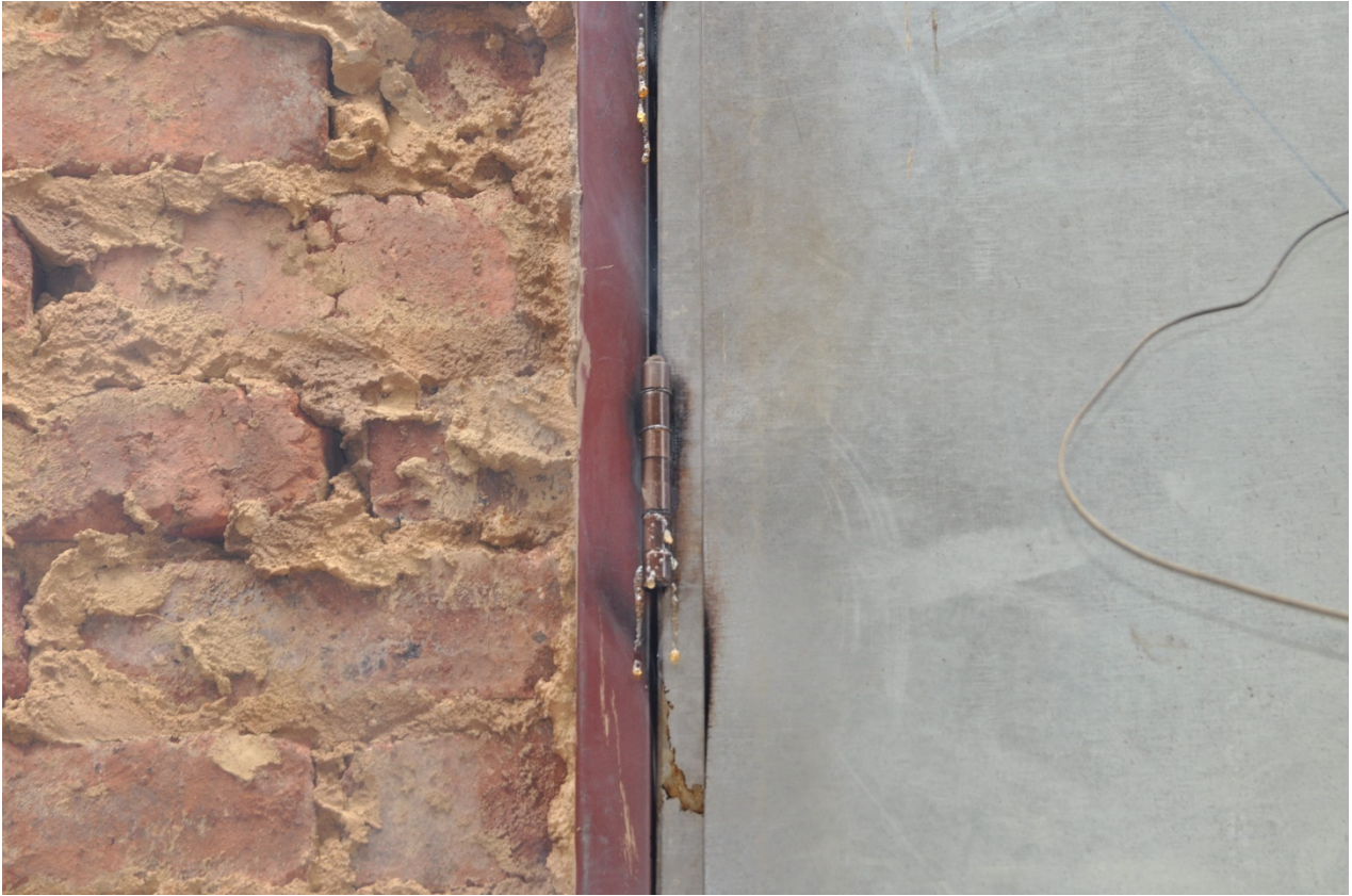
Figure 4.2.7: Hinge washers melting
