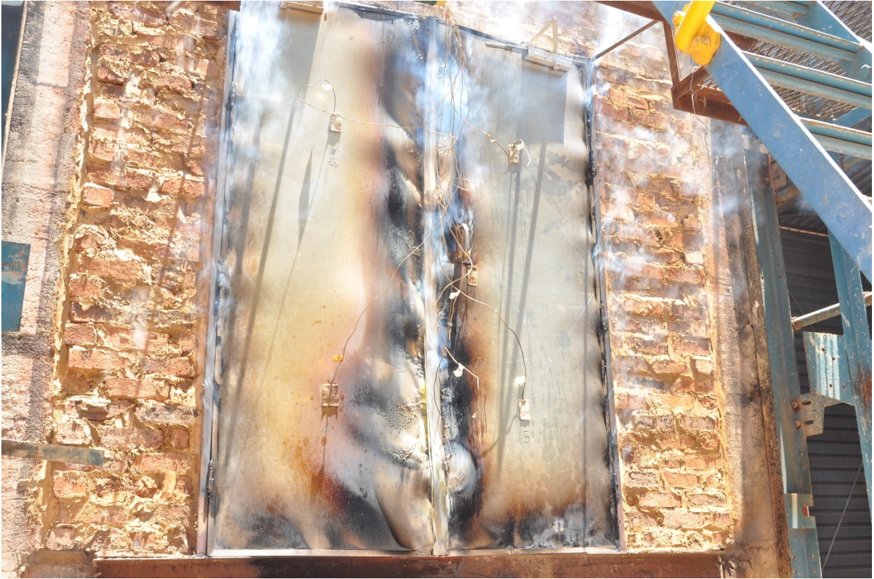
Figure 4.2.9: Door facing warping at 2 hours
