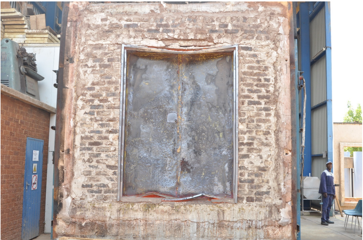
Figure 4.2.10: Exposed side of specimen at conclusion of the Fire Resistance test
