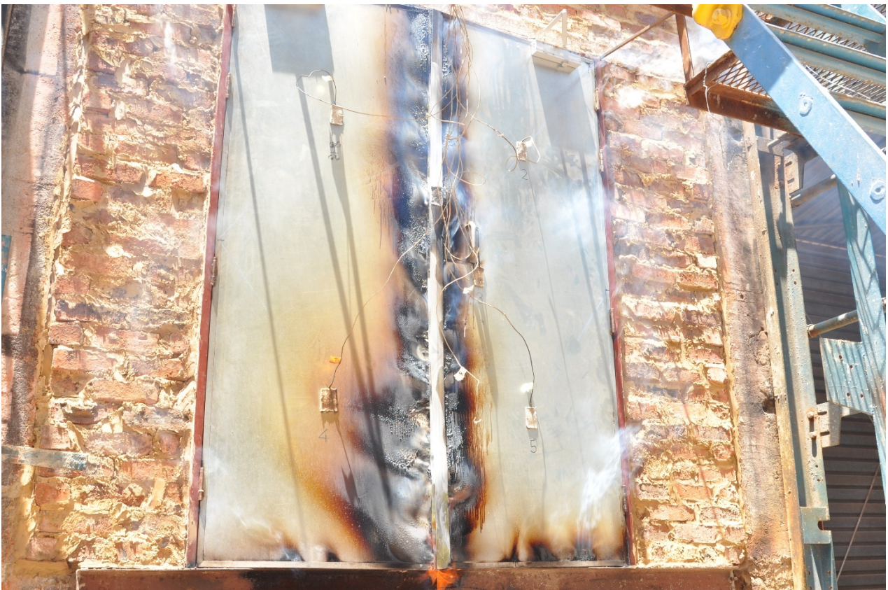
Figure 4.2.6: Door facing warping
