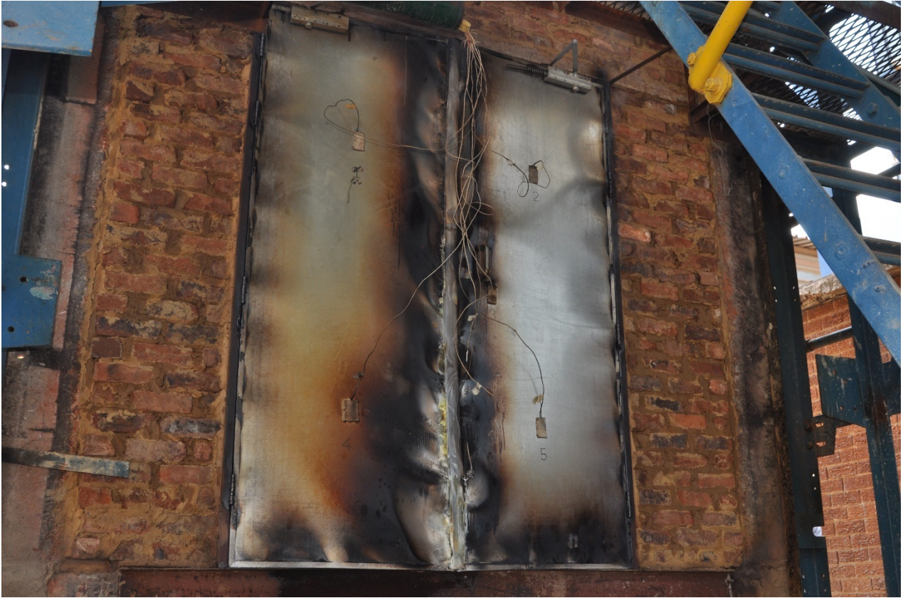
Figure 4.2.11: Unexposed side of specimen at conclusion of the Fire Resistance test
