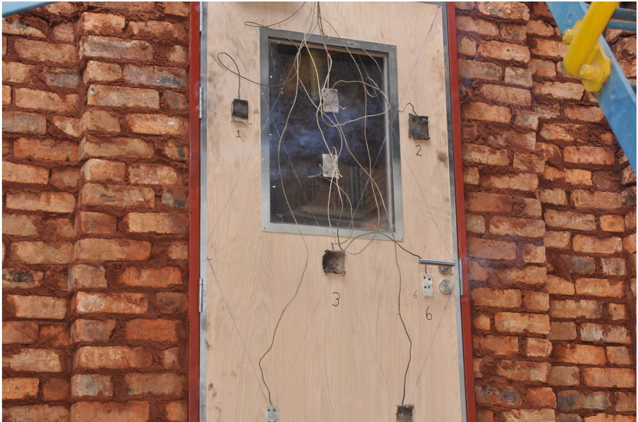
Figure 4.2.3: Light smoke release from left and right perimeter
