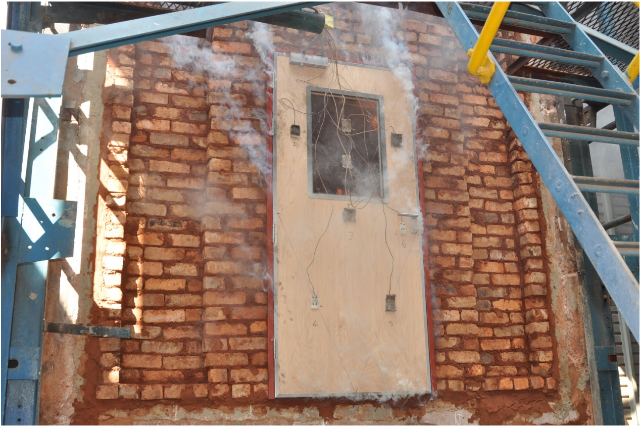
Figure 4.2.5: General smoke release increase
