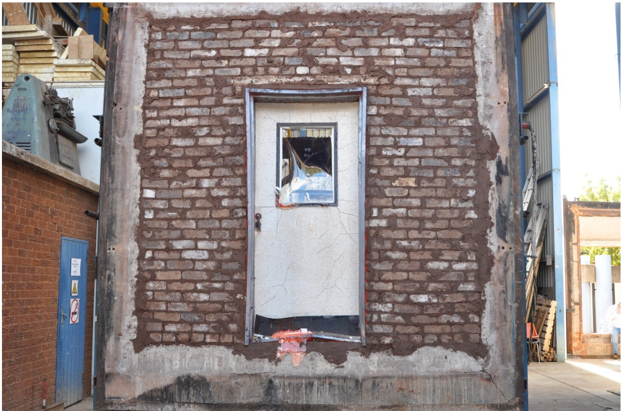
Figure 4.2.20: Exposed side of specimen at conclusion of the Fire Resistance test
