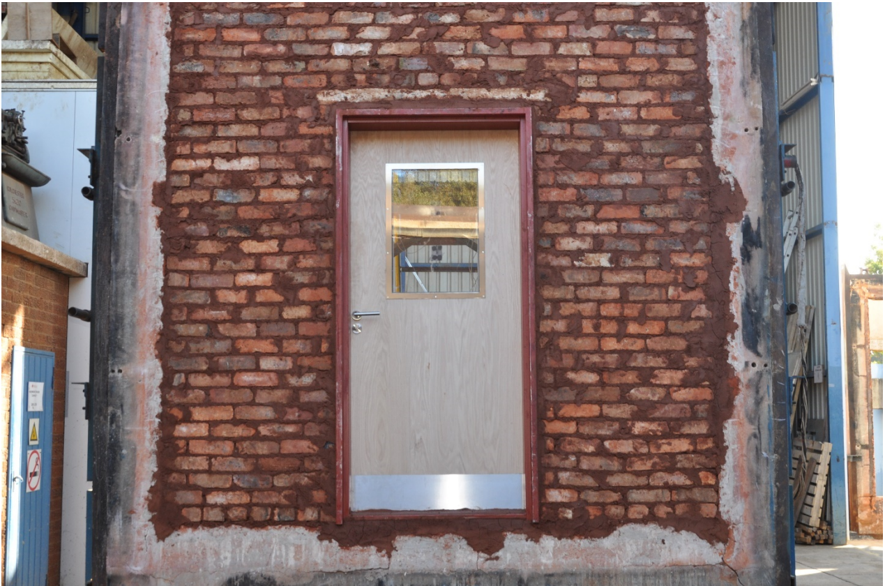
Figure 2.1: The 452 Glazed Door from the exposed side prior to the test
