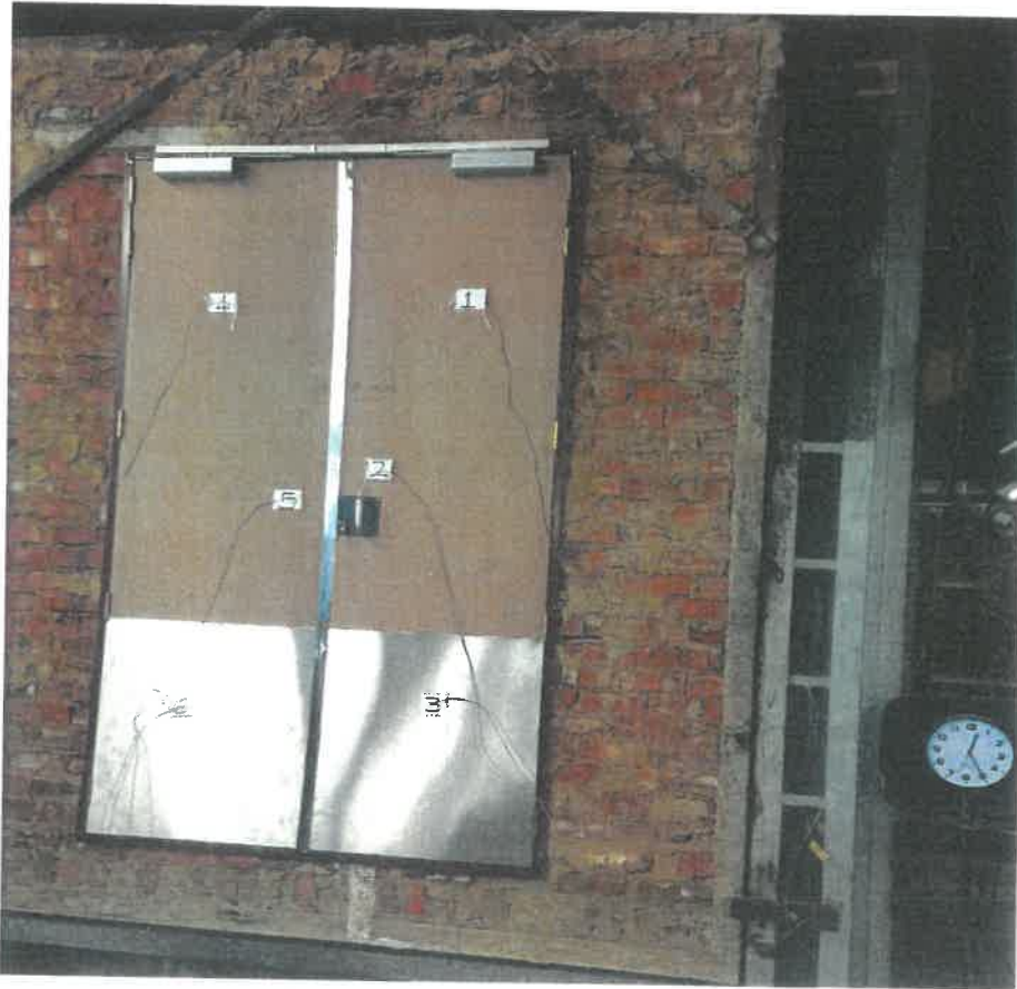
Photo 5: At 25 min, door still intact
