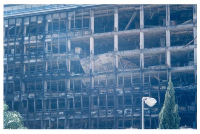
P&H Fire Seal Exposed to Fire for 24 Hours – P&H Seals still Intact even though the steel was exposed.
