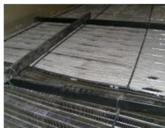
P&H Rocklite 'GC' 2 Hour Fireproof Ceiling, Top View of Rocklite 'G' Plaster and Riblath Sheet.
